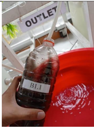
Sampling Outlet Treatment Lengkap
