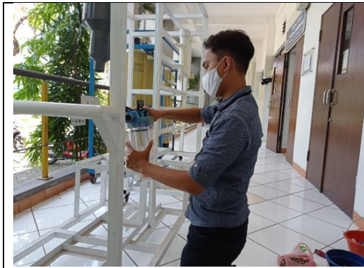
Pemasangan Housing Filter Kosong
