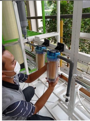
Pemasangan Housing Filter Resin
