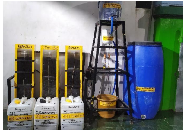
Gambar 10. Running Pengolahan Air Limbah Laundry
